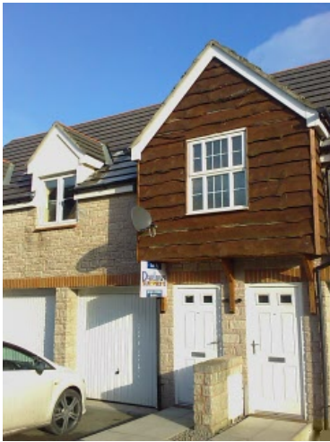
Front of building
